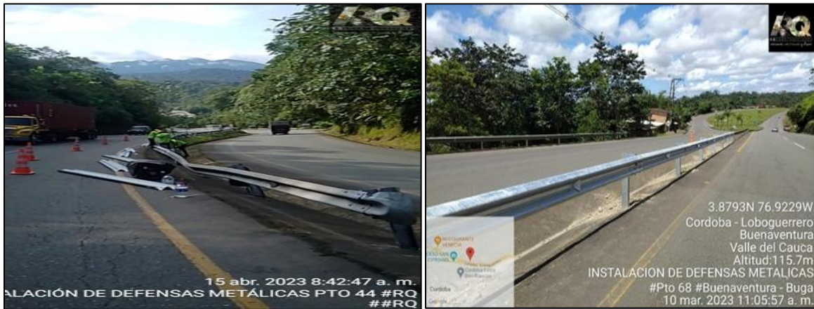
RN 4001 – PR 26+860 Córdoba – Zaragoza – New Jersey
